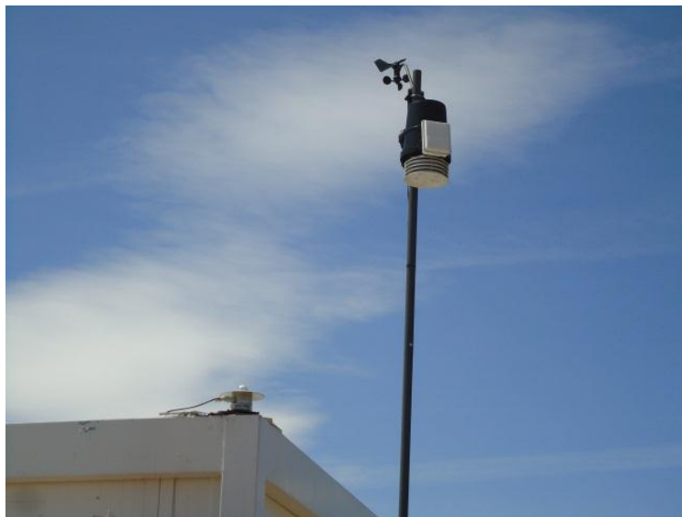
Figure 20 Weather station (on the left) and Pyranometer (on the right), located at the roof of Madrid DEMOPARK shelter.
