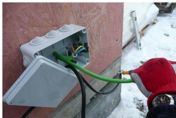
Figure 2 Electrical fitting-out at NANOPCM Mock-up.
