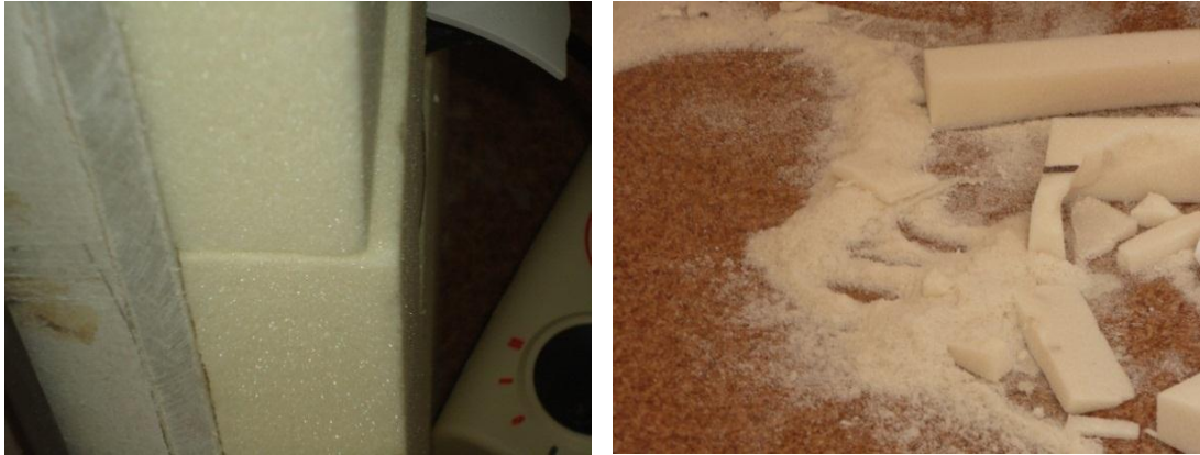
Figure 11 (left). Differences in size between NANOPCM panels. (right). Dust come-off the walls after installation.
