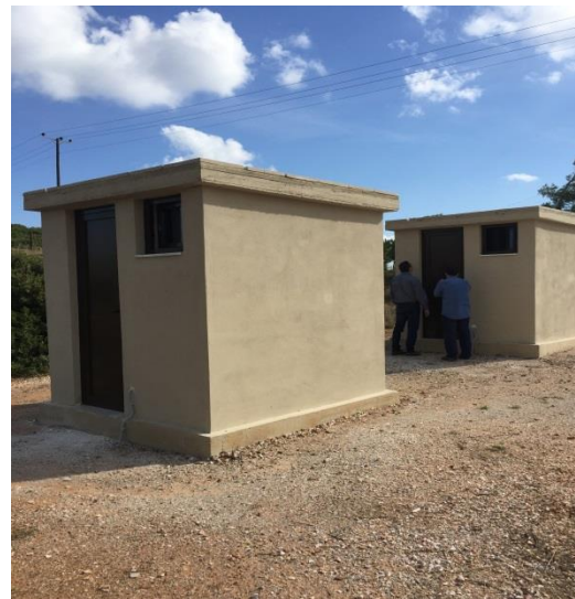
Figure 88: Final constructed buildings for monitoring
