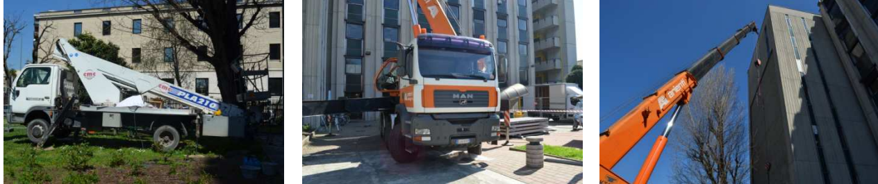
Figure 14: Equipment for panels installation
