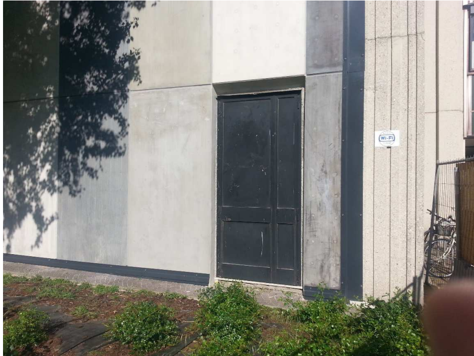
Figure 16: Test facade installed
