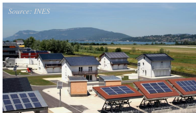
Fig.3: Experimental platform located at the French National Institute of Solar Energy (INES) near Chambéry / France. The experimental platform is used for testing novel materials and systems, e.g. by the EU funded HOMESKIN project ( https://homeskin.net/ ) in their development of thinner insulation systems and by other EU-funded projects
