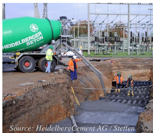
Fig. 1: Powercrete®, a high performance heat conducting concrete used for HV and UHV underground cabling to improve energy transport and distribution
